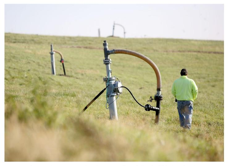
Dane County plans to continue extracting gas through a series of wells installed in its landfill, but instead of using it to generate electricity it will soon sell it through an interstate pipeline.
