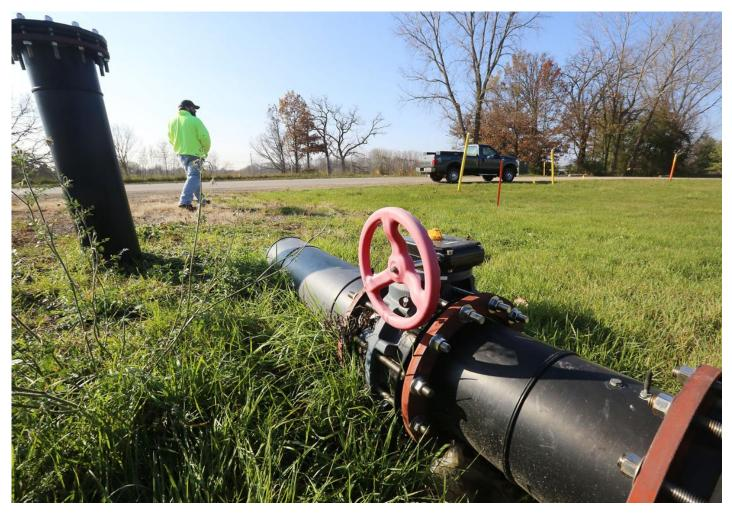
Dane County's landfill collects gas and pipes it to on-site electrical generators. A small amount is processed for use as automobile fuel. Plans are under way for a larger processing facility to prepare the gas for sale through an interstate pipeline. JOHN HART, WISCONSIN STATE JOURNAL
