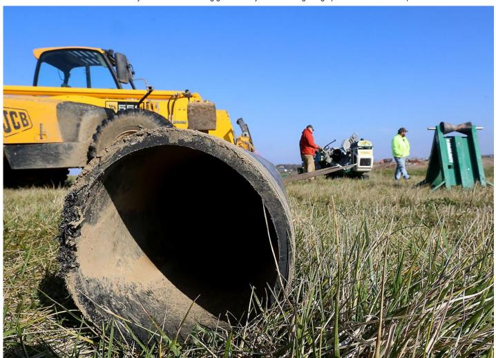
As the Dane County landfill prepares to begin selling gas through an interstate pipeline, it is installing other pipe to collect gas from a new landfill section.
