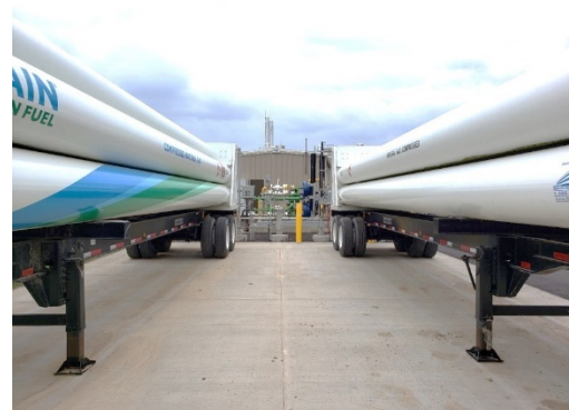
Biogas is produced at Wisconsin digesters and brought to the offloading station for injection into the pipeline.
